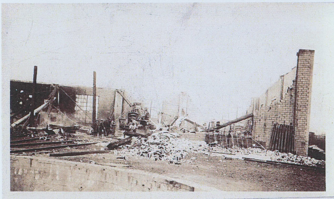
Nothing was spared including the shop area.
