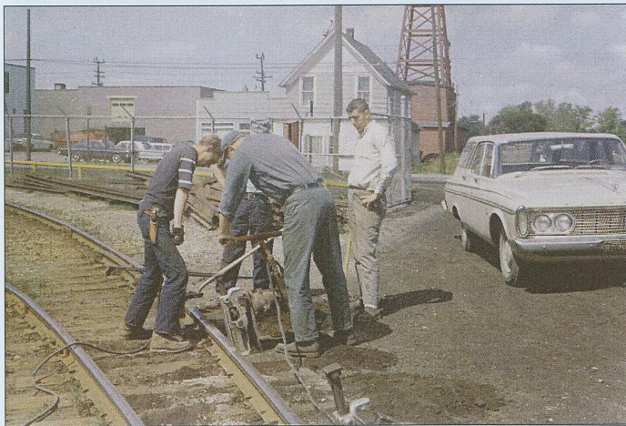
Section gang tamping a newly-replaced outside rail.
