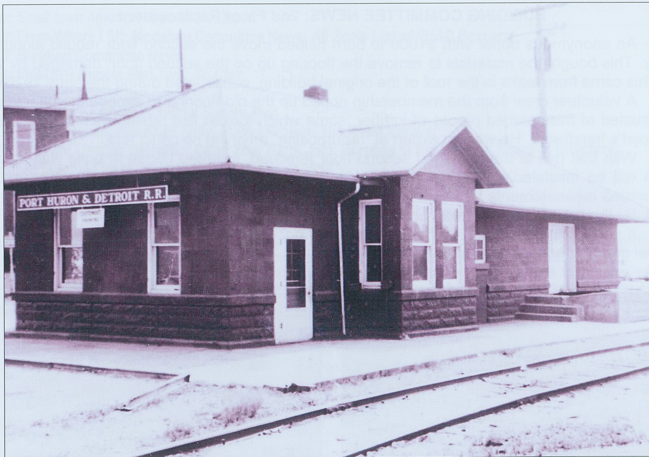
The two different cement block styles are evident in this late 1960's shot. An REX sign is displayed in the far left window.
