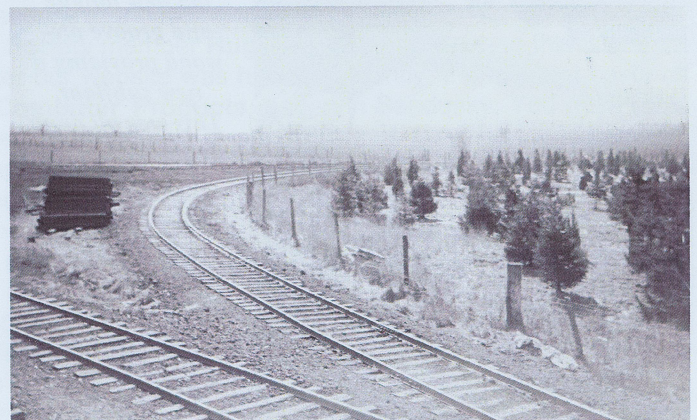
The wye extended west to allow a south-facing steam locomotive to head back north.
