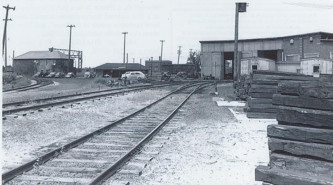
Employees entered the wye yard from 32nd Street, passing by the exposed concrete turntable foundation. Four tracks from the roundhouse shrink to one as they pass "The Reefers", 36' conversions occupied by Roundhouse Foreman Nate Georgian and his wife. On the right, concrete foundations from the steam era still remain under those ties. (Photo: Duffy Collection)
