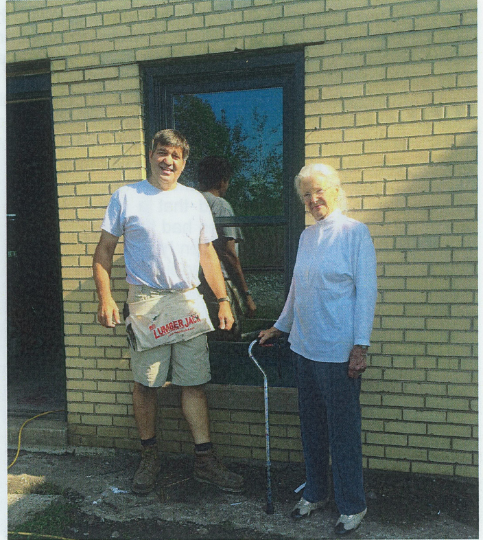
Kay Houghton with installer Tom from Shoreline Windows and Doors
