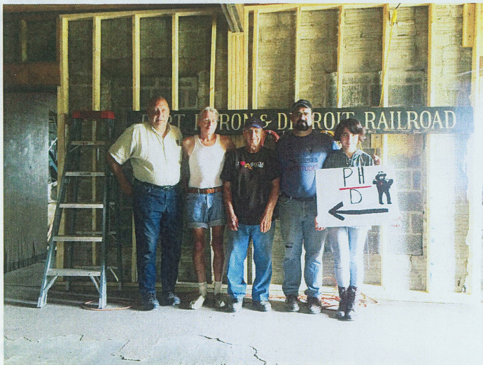
The Wiring Crew (LtoR): Dave Schultz, Dave Kennedy, Bruce Sawdon, T.J. and Phoebe Gaffney
