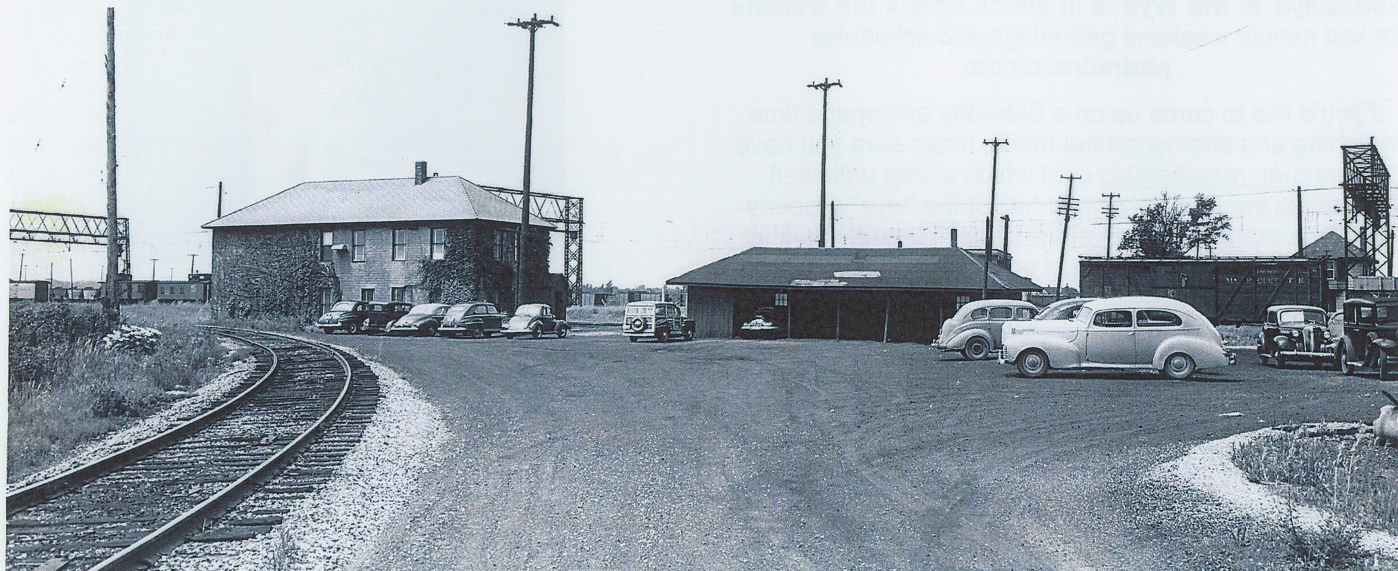
On the right, the rim of the turntable is totally exposed. The pit has been used as a catch-all for miscellaneous material. Employees drove into a cinder base parking lot. The two story office still looks the same today. For modelers, this scene has many transition-era details of the postwar years. That west leg wye curve looks nicely "dressed" eh? (Photo: Duffy Collection)
