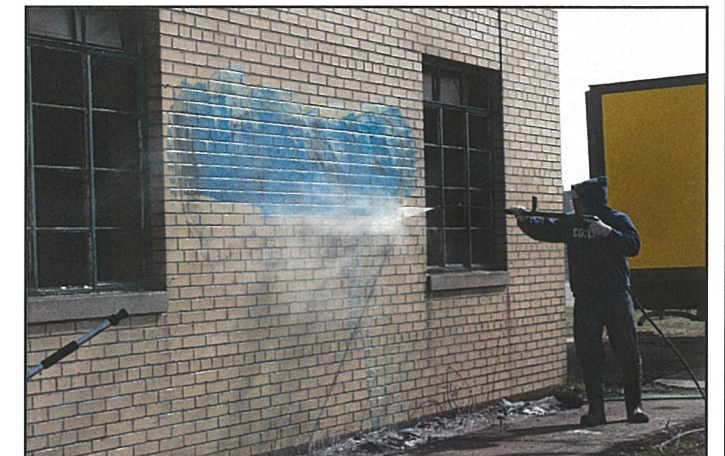
Blasting away at graffiti
