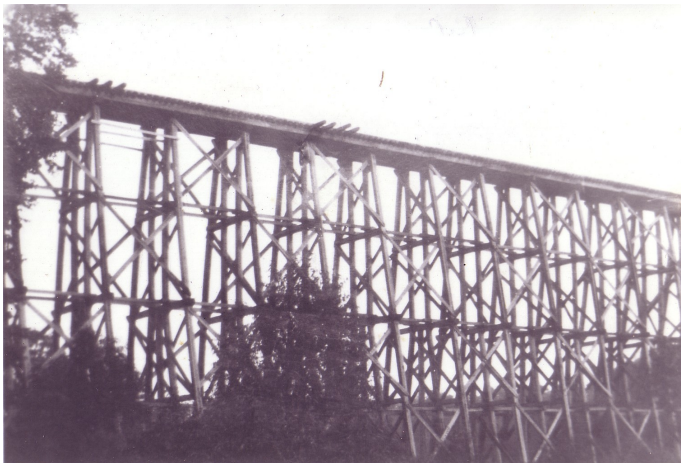
DBC&W Mill Creek Trestle Built by William Boyd, Chief Engineer DBC&WRR
