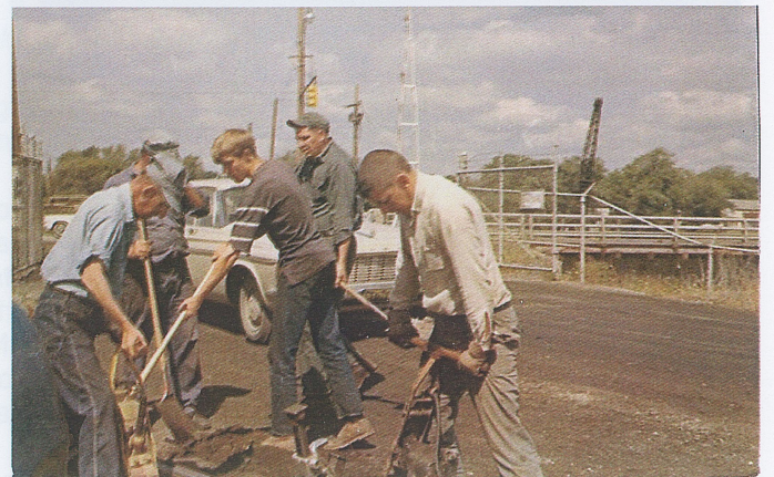
Bob Goulet (L) and Fred Witter (R) lean on the pneumatic tampers as Sandy Duffy, and Bill Parneski feed the gravel.
