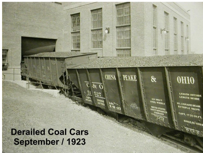
C&O #52527, built in 1909, has a capacity of 55 tons. It, and MC #11389, will need some serious blocking and jacking.
