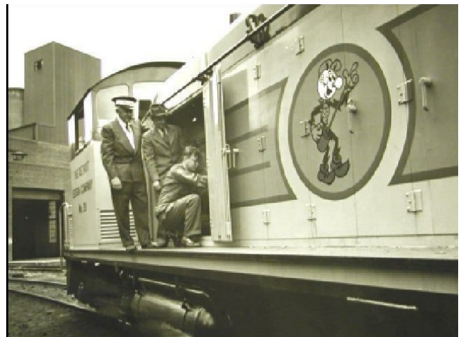
Here's Reddy Kilowatt who many of us remember on this company switcher.
