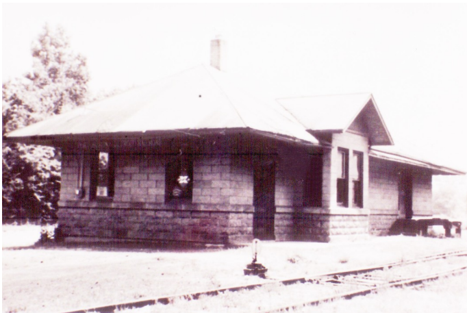
The depot window advertises that we're an authorized REX shipper. The switch leads to Reed Products. And there is that loading dock Doris referred to. Just leave a boxcar there for loading and pickup the following day!
