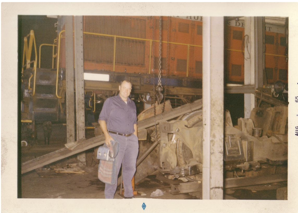
George Redfield has arrived with lunch bucket in hand, having been pulled from the section gang. The side frames are exposed and the crane stands ready to hoist them to expose the wheel/tire assembly.
