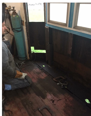
The bay window exposed.
