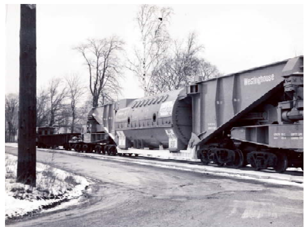
This Generator-Stator required a custom flat from Westinghouse with 20 axles, 10 on each end.
