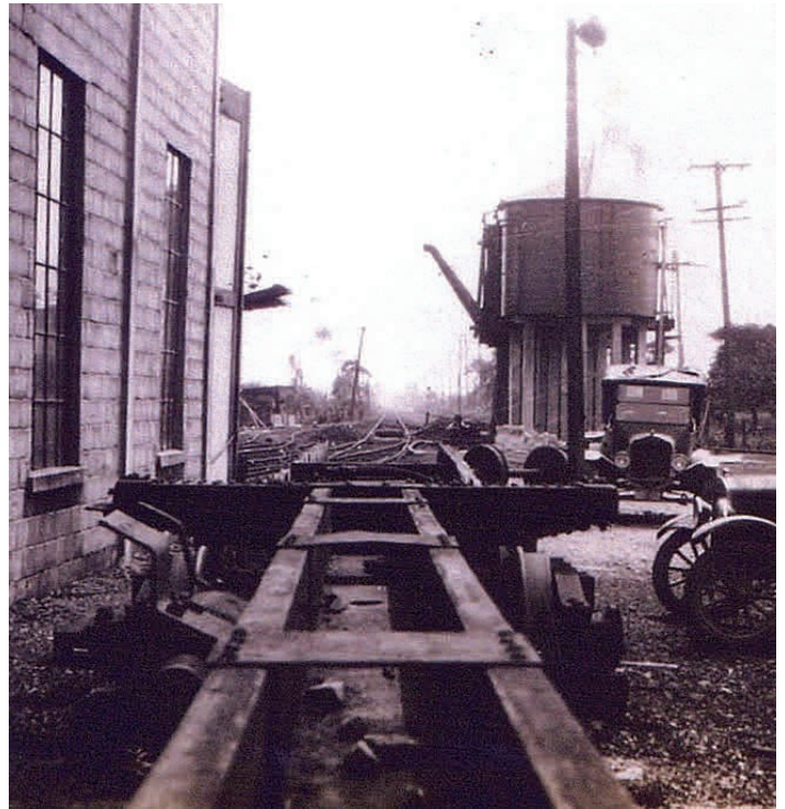
In this ca. 1930 view looking south, we can see the two water plugs. By now, the original roundhouse wall has been enlarged, hence the close proximity of this spur. The coaling chute is visible just beyond the open MOW door and in the distance, we see that same high mount switch stand.
