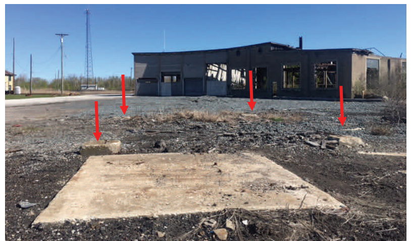
Four coal tower foundations with sand house slab.
