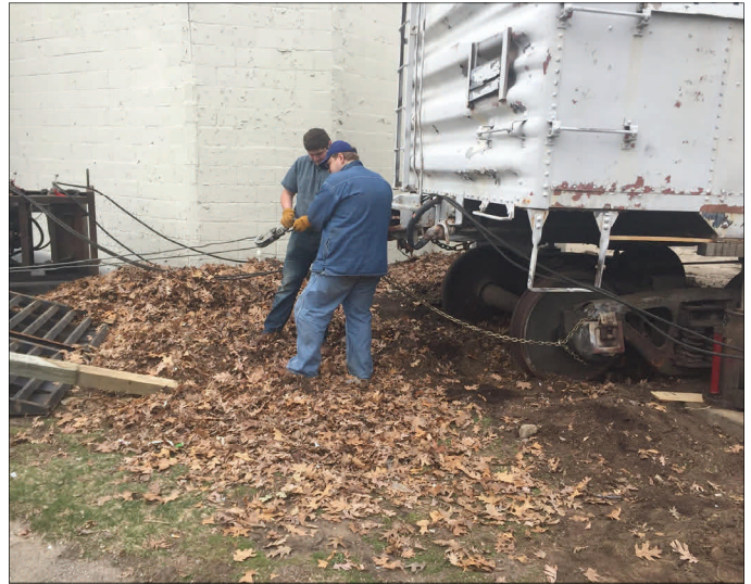
With the GTW reefer on jacks, Judd Brown (facing) and Society board member Chad Thompson prepare to remove the first set of trucks.
