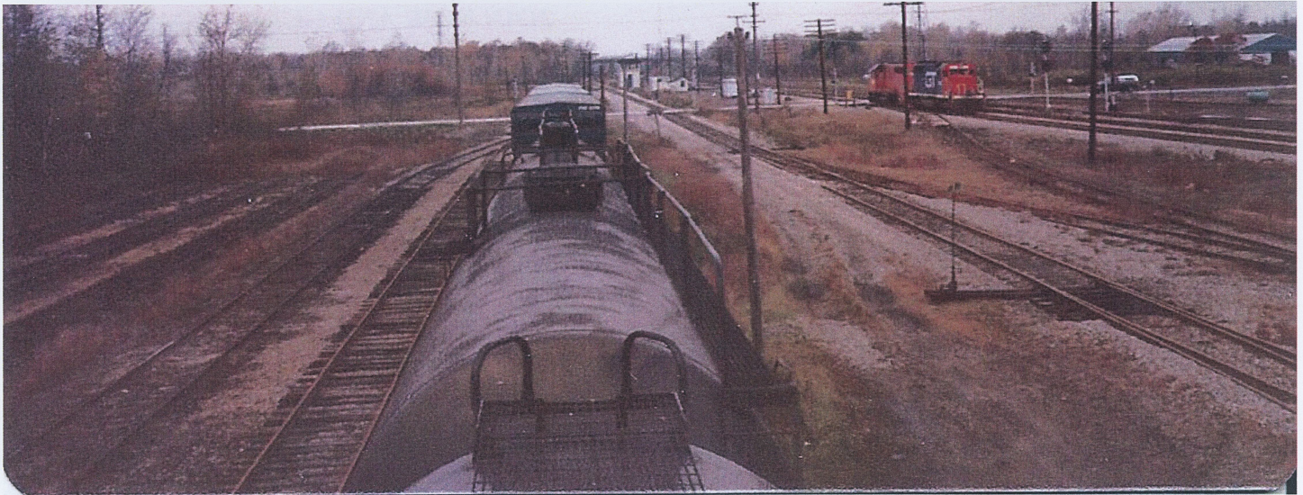
Then: On the left, runaround Tracks 1 & 2 curve into the main while numbers 3, 4, & 5 are stub ended. On the right, is the PM/C&O interchange with the GTW. Their transfer track with the PH&D begins with that switch on the right.
