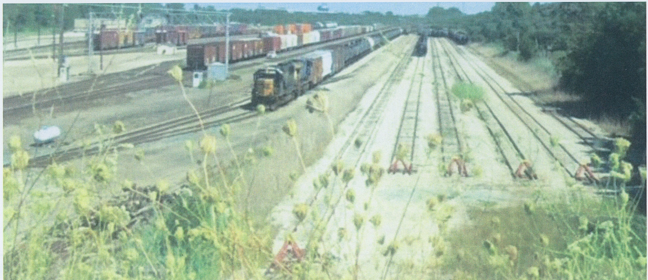
Now: A CSXT train waits to run west on the GTW main. All yard tracks have been converted into stub end sidings removing the old PH&D/Grand Trunk interchange. The access road in the middle remains but gone is the PM transfer track.
