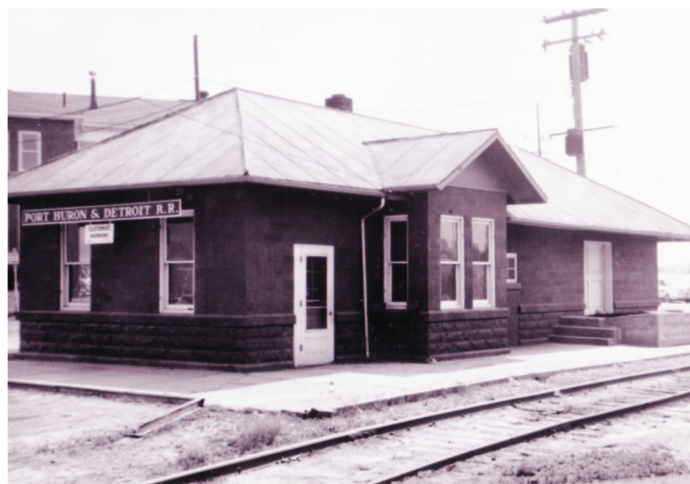
St. Clair Freight Station. The loading platform on the right corner slants up to a level matching the height of the average boxcar floor. A back room contained weighing scales and packaging materials. Barely visible is the red and white "REA" sign in the window on the far left, under the station sign. This station sign is in our possession.
