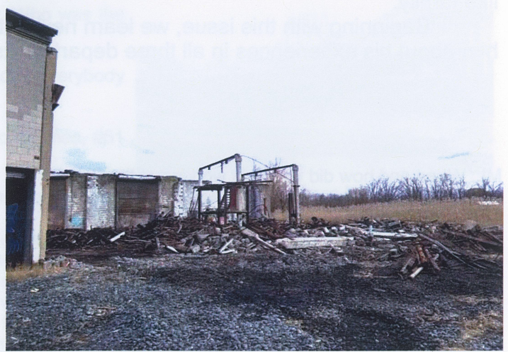
It's December 2018 and all walls of the original structure have been razed except for the north wall. (Photo: William Rauli)
