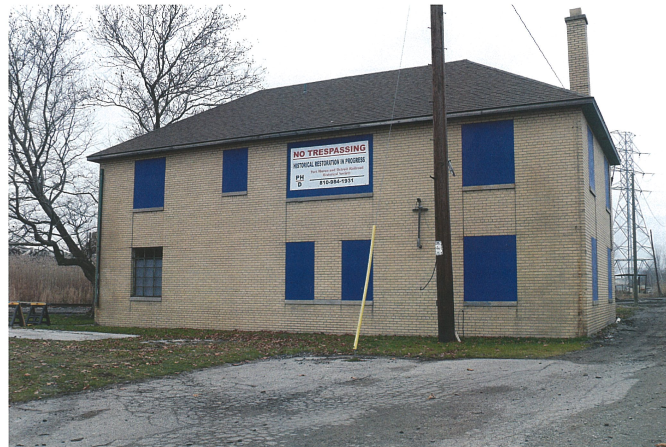
All windows are boarded up except for the corner Agent's Office which will receive windows. This will be our temporary office!
