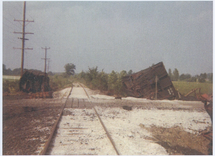
Looking north. The priority was to first remove the cars, then get the main clear for revenue operation.
