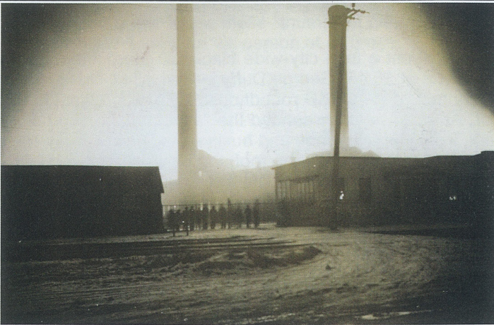
13 cars loads were totally destroyed along a loading dock next to the banks of the St. Clair River. This image is of a loading dock next to the River road. It too would be consumed.
