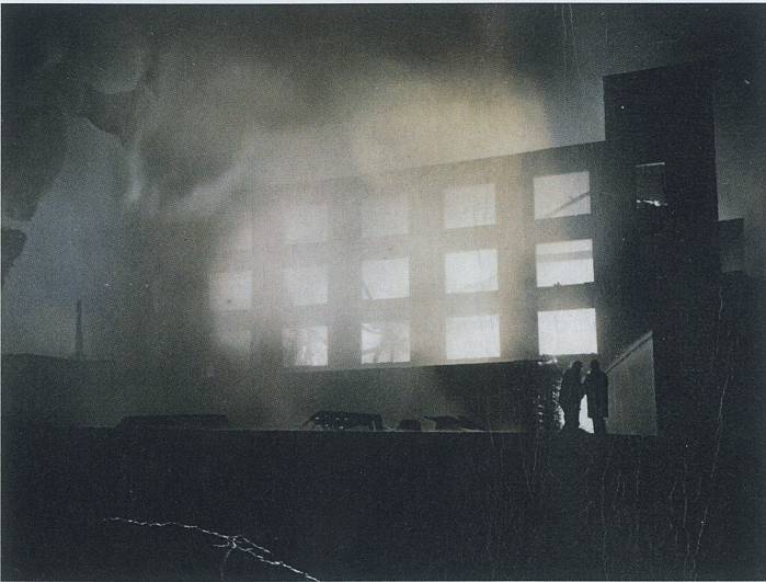
Of the 18 buildings, only 3 remained relatively untouched. This 5-story dairy mill would be gone in a matter of hours.
