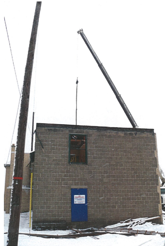
Brand new roof trusses next to the office await placement as the crane pulls off sections of the old roof.
