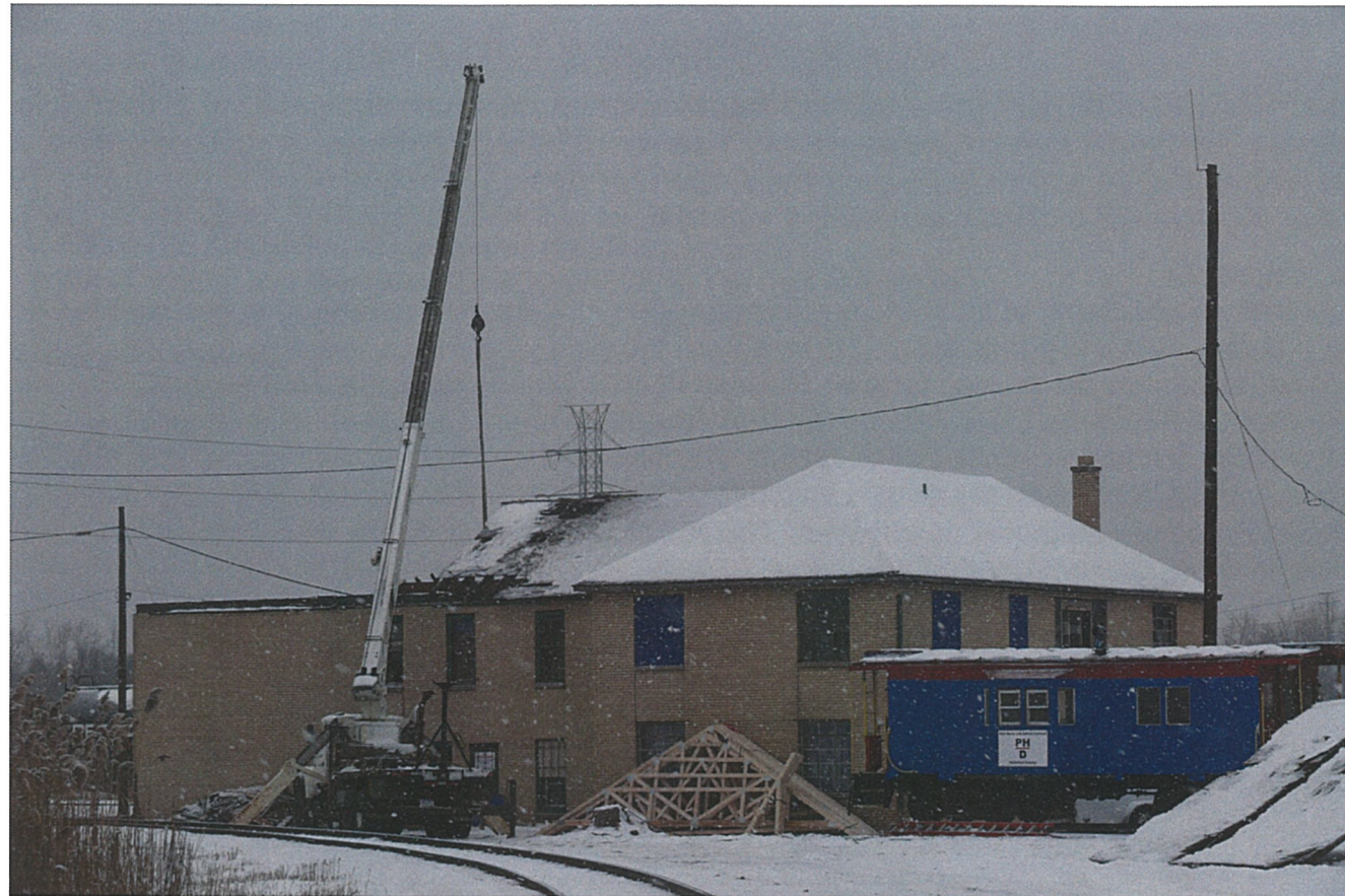
Brand new roof trusses next to the office await placement as the crane pulls off sections of the old roof.
