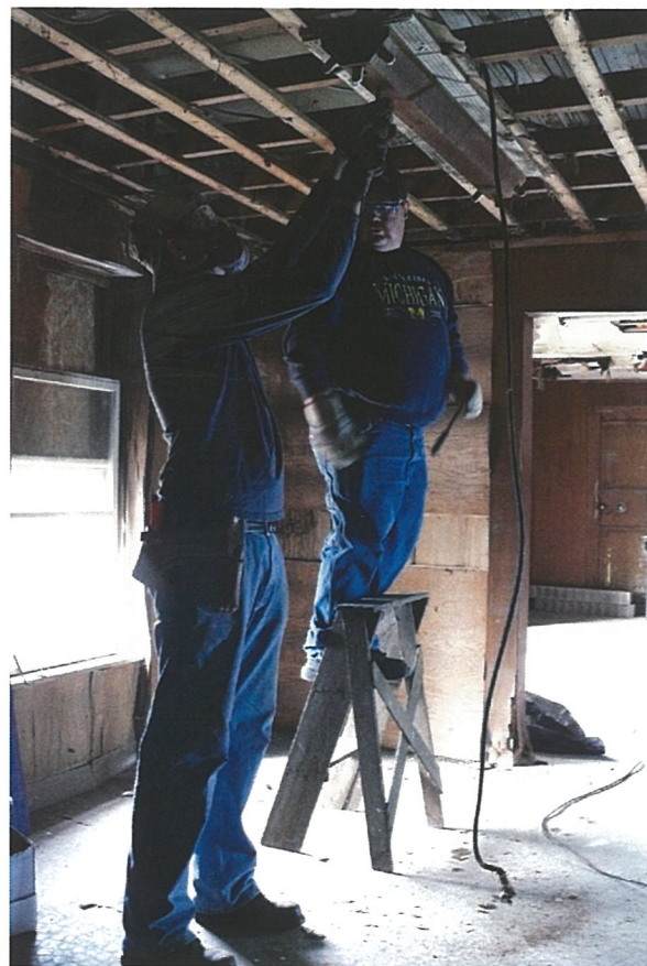
Charley Warsinski and Dave Cenci removing an office light.
