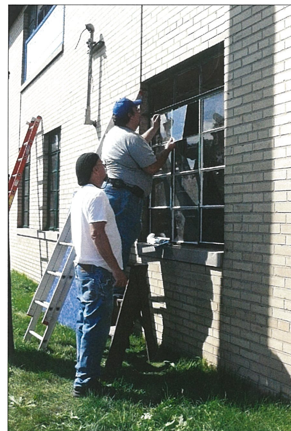
Glassman Don Burton watches Tom Grambau insert a pane.
